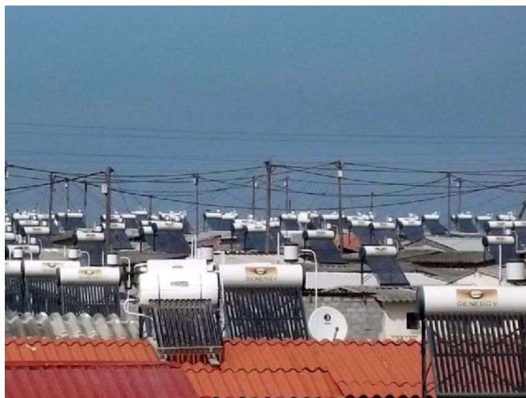
Solar water heaters on homes in Kuyasa, South Africa, installed as part of the CDM project for the township. (Source: https://energygeographies.wordpress.com/south-africa/ )
